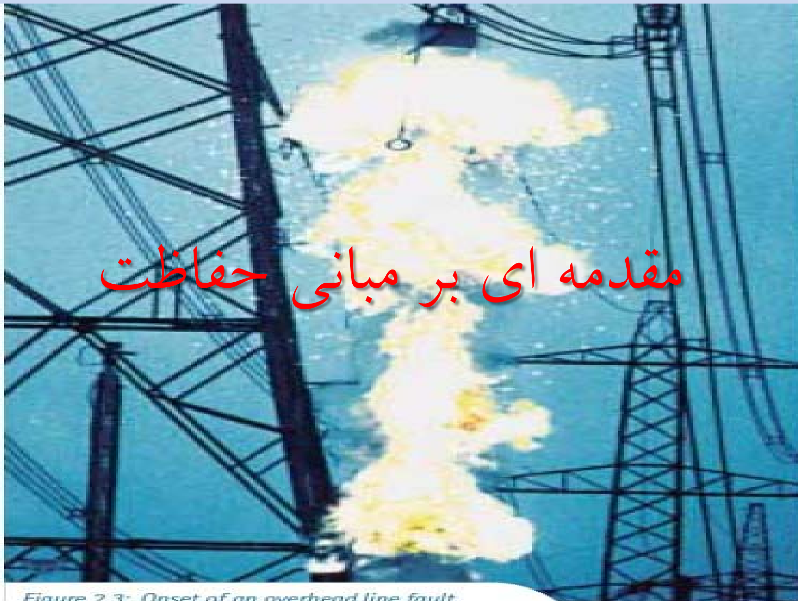
Figure 2.3: Onset of an overhead line fault.
